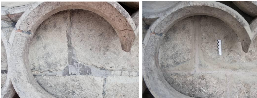
Fig. 3: Cologne, Cathedral, Window S 3, wall area in tracery, before (left) and after (right) restoration © Dombauhütte Köln / photo: M. Unkelbach
